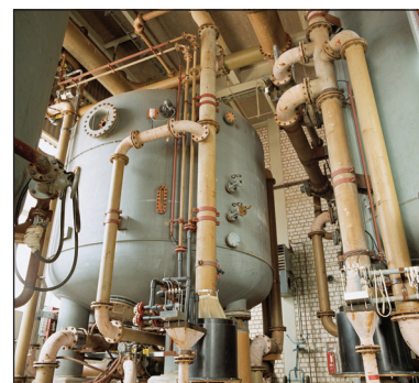
Figure 3: The removal of chemical substances in trace quantities can be carried out by means of additional filters that are equipped with selective filter materials
